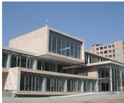
PflD's new learning center opened in 2012 and has approximately 24,000 square feet of space.
